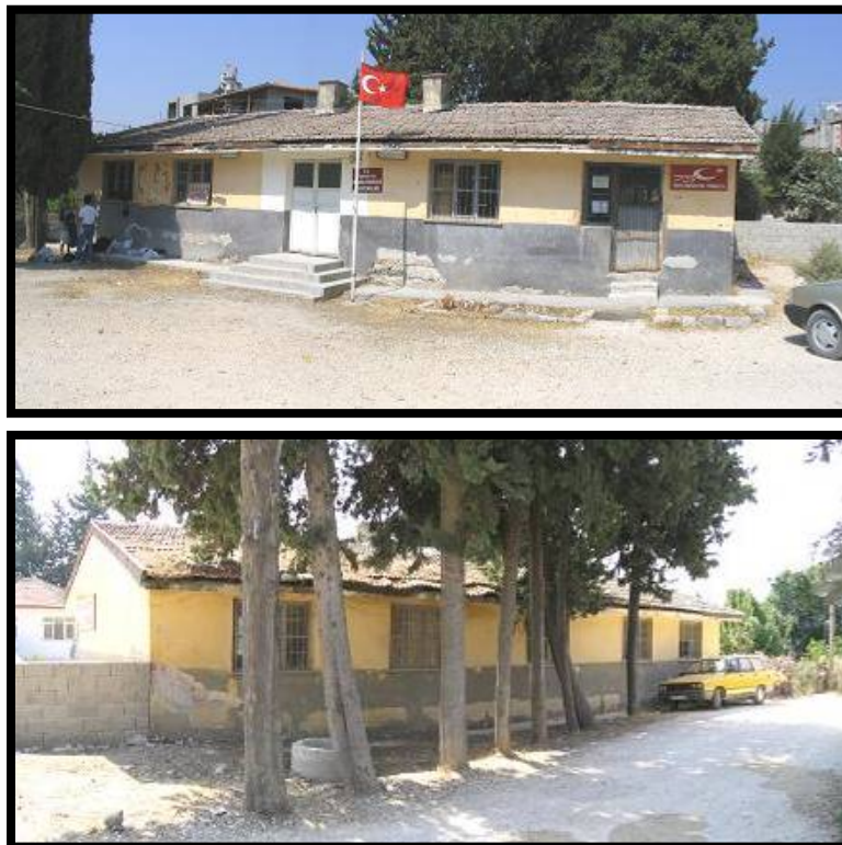
Figure 1 General view of the evaluated single storey URM house
