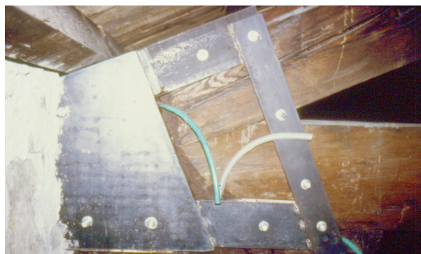
Figure 3 – Overstrengthening of a carpentry joint
