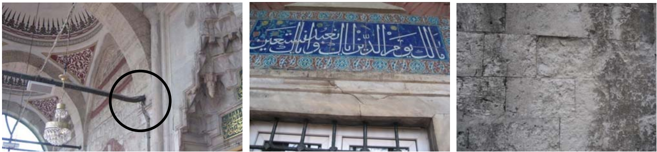
Figure 3 Observed damages
