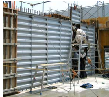
(a) Use as webs of a bridge (b) Use as a shear wall in a school building Figure 4 Practical uses of corrugated steel shear panels
