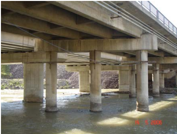
Figure 4 Old bridge with 3 column bent
