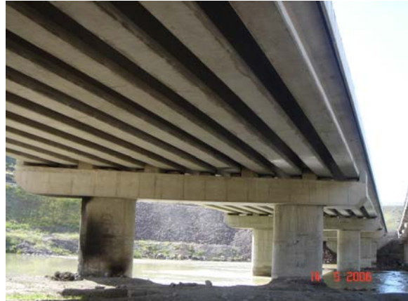
Figure 5 New bridge with 2 column bent
