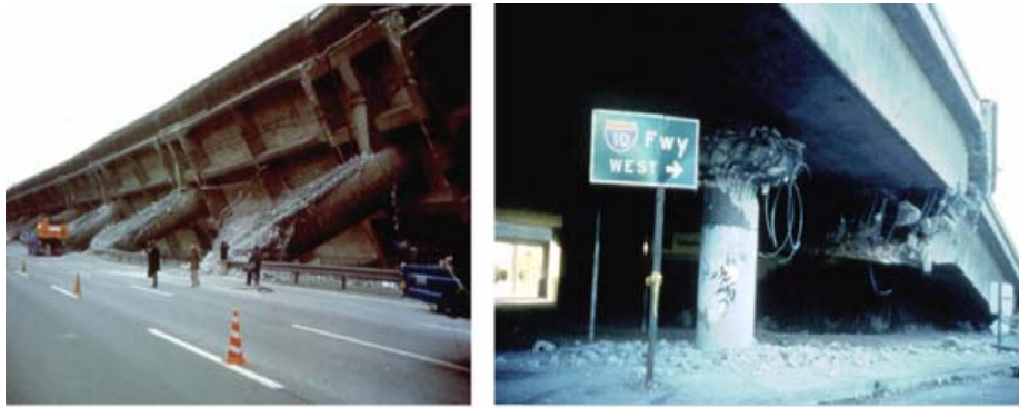
Figure 1 Damages observed to bridges (Riobóo, 2005)
