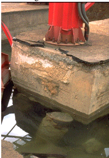
Fig3~4. detachment failures between pile head and pile cap, Higashi bridge, Hyogoken-Nanbu earthquake
