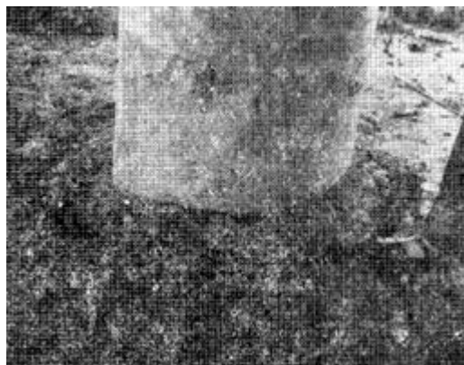
Fig 2 Gaps with differential wide opened around the piles, Tangshan earthquake
