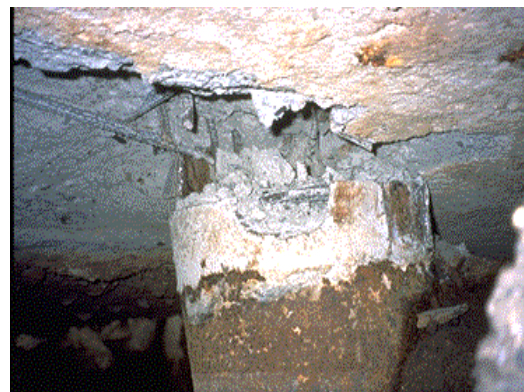
Fig3~4. detachment failures between pile head and pile cap, Higashi bridge, Hyogoken-Nanbu earthquake
