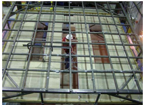
Figure 15. Specimen II at test completion
