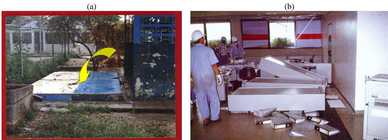
Figure 6. (a) Overturning of masonry walls and (b) Overturning of shelves (MIDAS, 1997) during the 1997 Cariaco earthquake.
