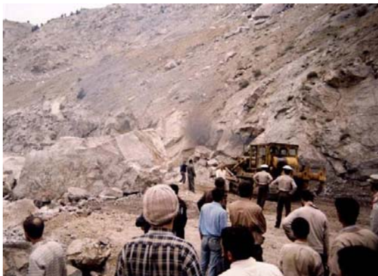
Figure 1 Damages to main roads caused delay in dispatching the search and rescue teams to the affected sites; (A) Rock fall in Manjil Earthquake (1990), and (B) Collapse of Qanats in Bam Earthquake (2003)
