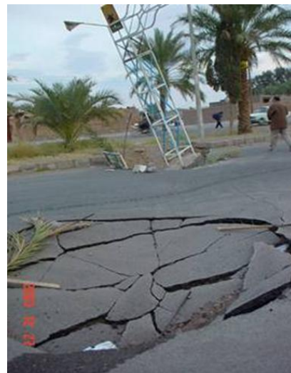
Figure 1 Damages to main roads caused delay in dispatching the search and rescue teams to the affected sites; (A) Rock fall in Manjil Earthquake (1990), and (B) Collapse of Qanats in Bam Earthquake (2003)
