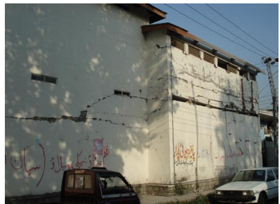
d) Unconfined brick masonry
