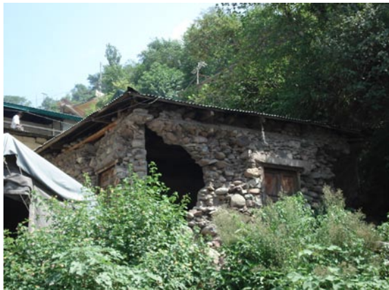
a) Stone masonry
