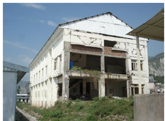
f) Reinforced concrete frame
