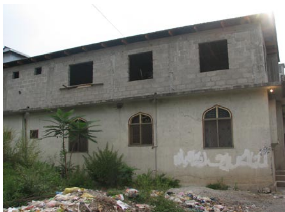
c) Concrete block masonry
