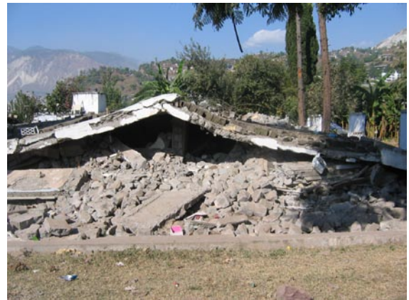
b) Unconfined concrete block masonry
