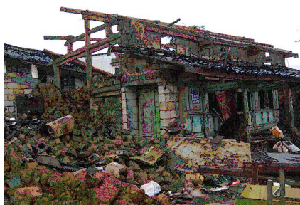
Figure 4. The house was destroyed in Pu’er earthquake
