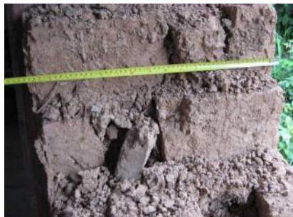
Figure 6. The earth wall with thickness of half meter
