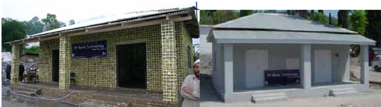
Figure 3: Retrofitted house in Pakistan before and after application of covering mortar layer 1
