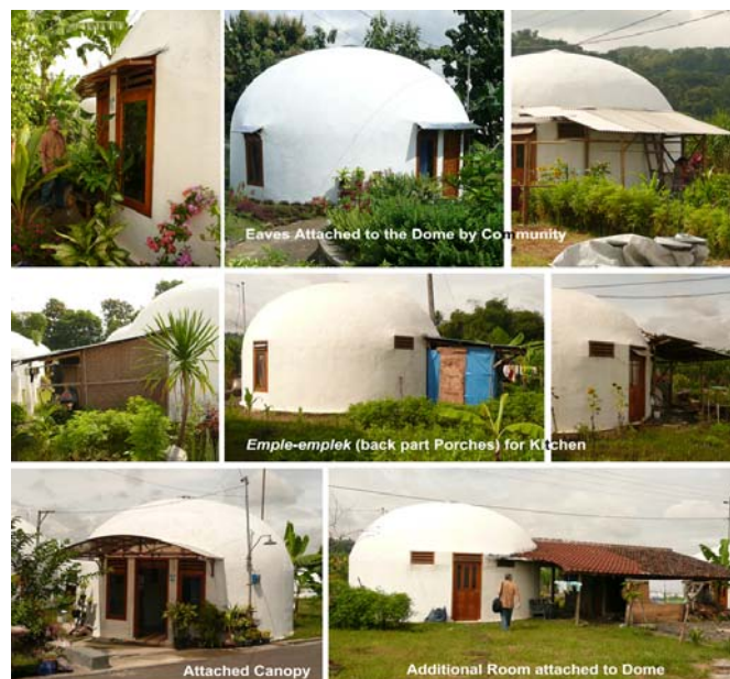
Figure 13. Additional Elements attached to dome by Inhabitants
