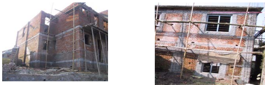
Figure 1 Earthquake resistant re-construction and retrofitting of school buildings
