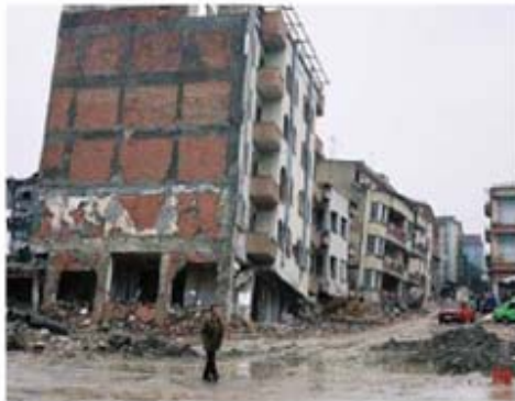
Figure 1. Many buildings failed in their ground floor during the Kashmir earthquake
