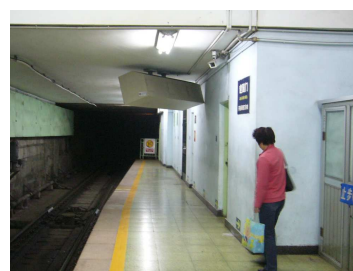
Fig. 8 No emergent refuge-exit in the Beijing subway station
