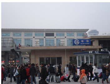
Fig. 2 Outside distinct of the station identification signs in Beijing subway station
