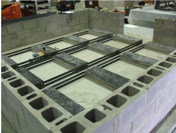
Figure 3 Concrete ball-in-cone isolators
