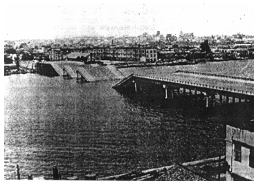
Fig. 2: Tangshan, China, 1976: Super-Structure Collapse
