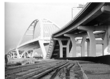
Fig. 6: Kobe, Japan, M=7.2, 1995: (Nishinomiya Harbour Bridge)
