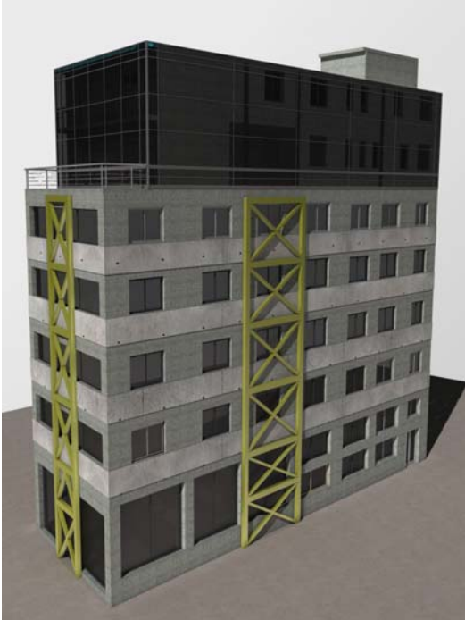
Figure 8: Building after strengthening
