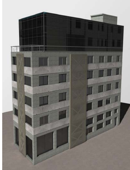
Figure 9: Building after covering of the strengthening
