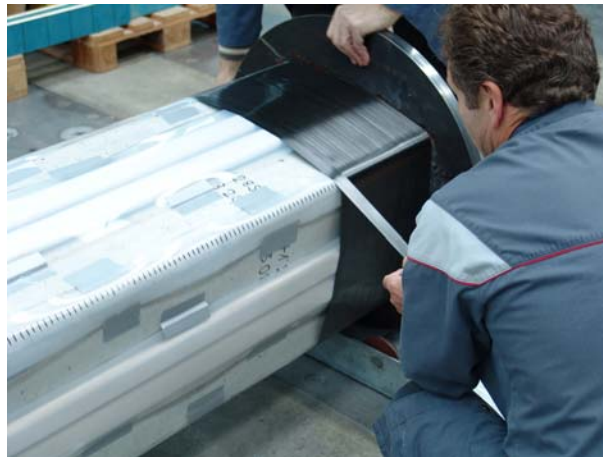
Figure 2 Wrapping of CFRP straps of column (3)
