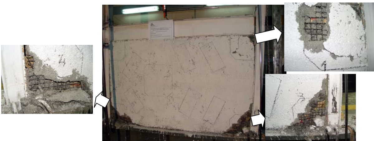
Figure 6 Retrofit side of the wall after test
