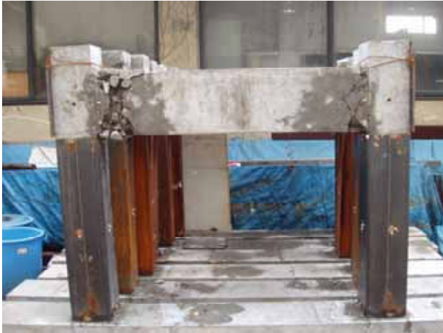
Photo 1 Frame with Normal-Strength Rebars
