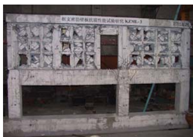
Figure 8 Failure phenomena of KZML-3
