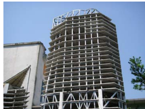
photo 5 the relative location of transfer story and upper-close column story
