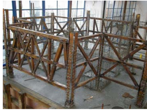
photo 3 consolidation of truss
