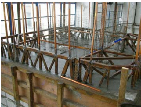
Photo 4 the connection of upper-close columns and truss
