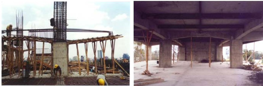
Figure 1 Typical RCHBs in buildings recently constructed in Mexico City
