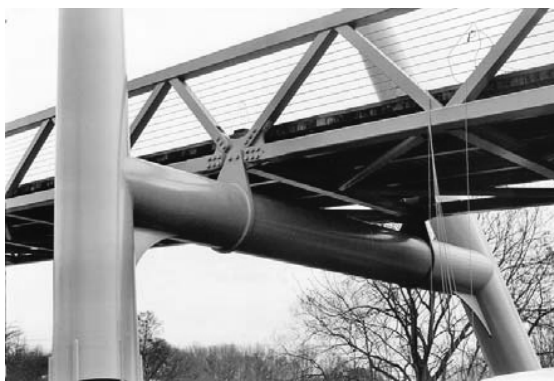
Figure 3 Connection girder-pylon
