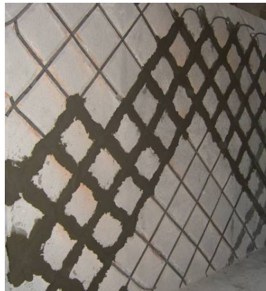
Figure 3. Strengthening by old tyre strips
