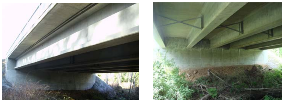
Figure 4. Millar Creek Bridge
