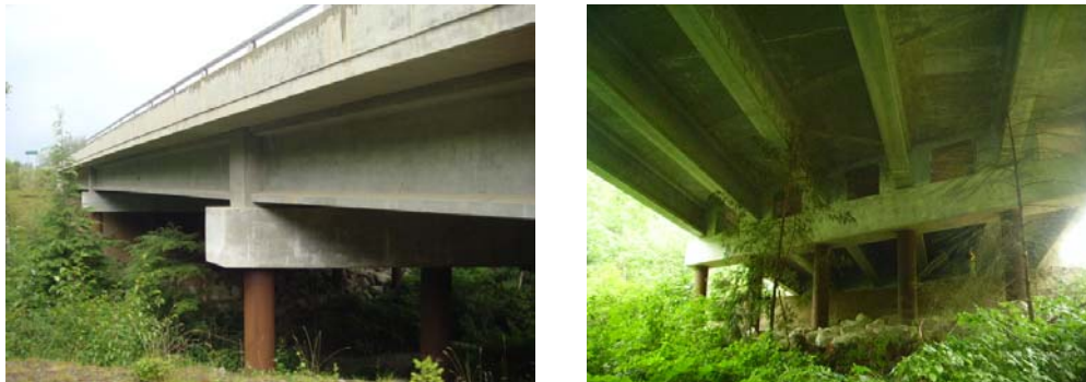
Figure 6. Black Creek Bridge
