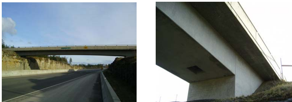
Figure 3. Duncan Bay Main Bridge
