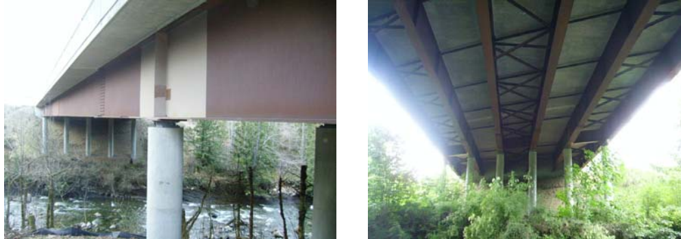
Figure 5. Browns River Bridge
