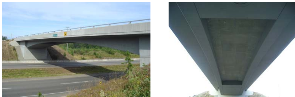
Figure 1. Royston Road Bridge
