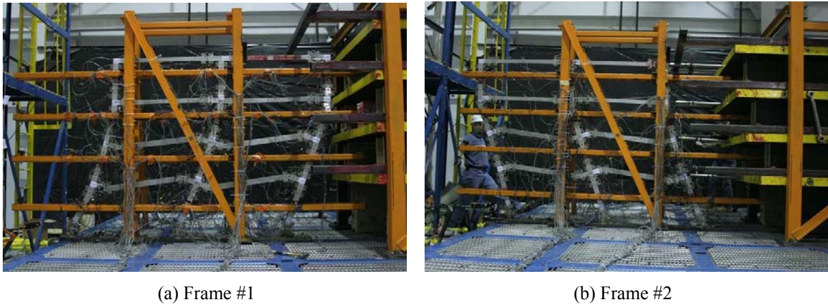
Figure 9. Collapse mechanism of both test frames after the completion of CLEF
