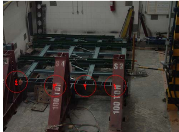
Figure 8. A frame of type I ready for test
