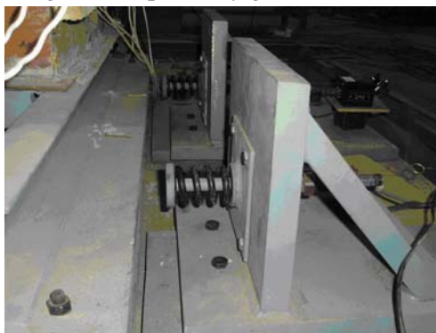
Figure 4 spring buffers installation
