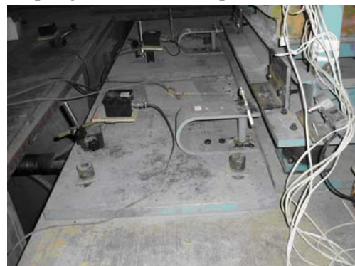
Figure 5 compound buffers installation
