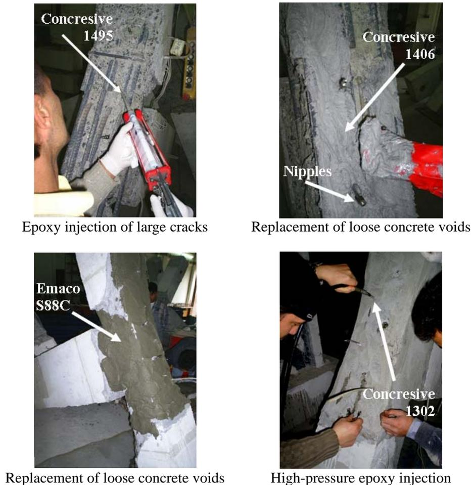
Figure 3.1 Repairing procedure
