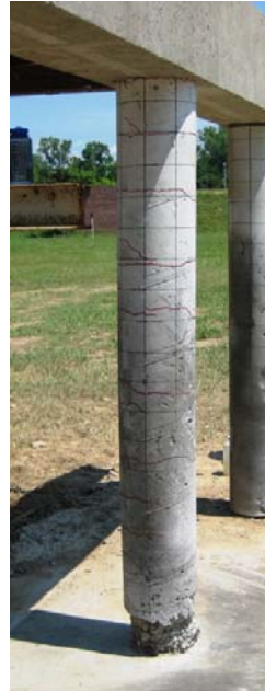
Figure 5 Column RC2 after test
