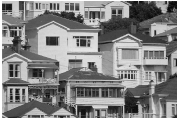
Figure 1: Wellington Inner Suburb.
