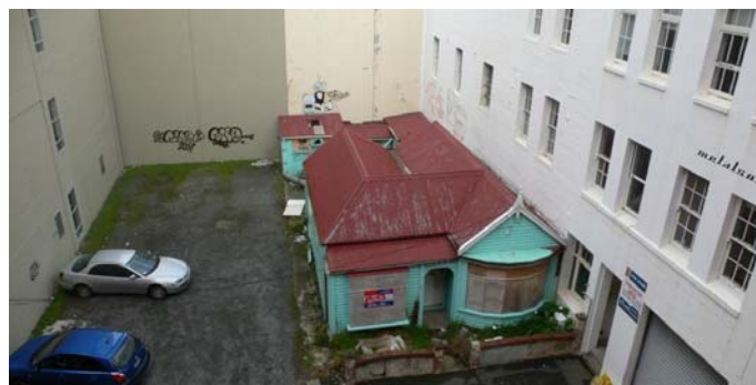
Figure 3. Buildings with unprotected roof and windows on boundary
