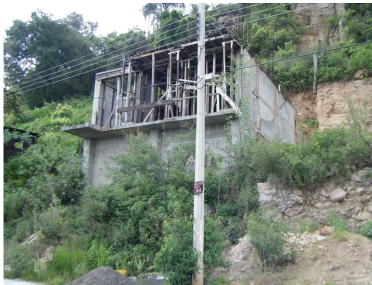
Figure 4 Construction on progress along the scarp (zone II)
