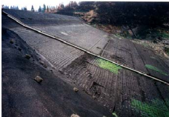
Figure 1 Damaged Kawanishi Dam (shallow sliding of the upstream slope, 2004 Mid Niigata Prefecture ) Earthquake)
