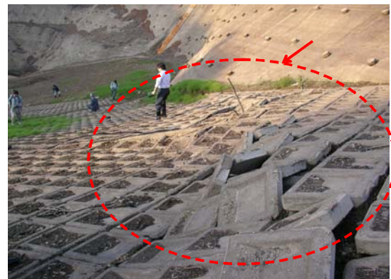
Figure 1 Damaged Kawanishi Dam (shallow sliding of the upstream slope, 2004 Mid Niigata Prefecture ) Earthquake)
