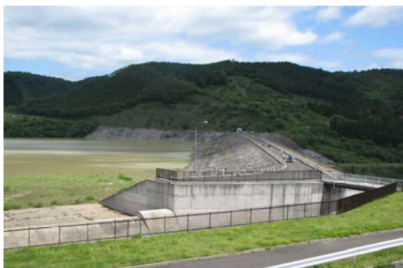
Figure 1 Damaged Kawanishi Dam (shallow sliding of the upstream slope, 2004 Mid Niigata Prefecture ) Earthquake)
