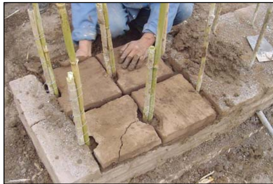
Figure 7 Appropriate bonding, rules as a main function for usage of the reeds as the tensile elements
