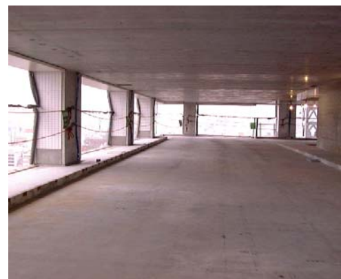
Figure 8 Inner Space under Construction
