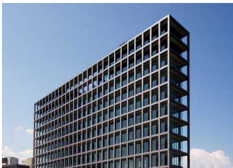
Figure 5: Façade on south side
