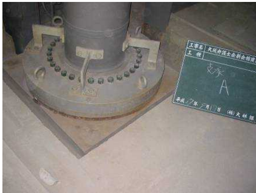
Figure 19: Appearance of pinned column plinth
