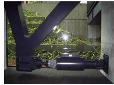
Figure 10: 1760 kN type oil damper
