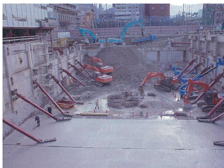
Fig. 17: Construction status of existing underground exterior walls to be permanently left
