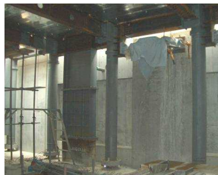
Figure 18: Hysteresis type dampers on intensive vibration control story
