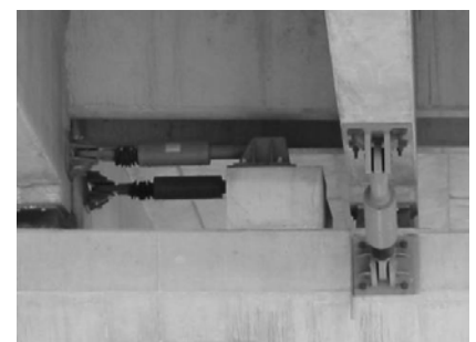
Figure 18 The 12 km long Rion-Antirion Bridge in Greece. The main bridge and its approaches were protected by SVPC devices manufactures in Italy (including 188 VDs).
