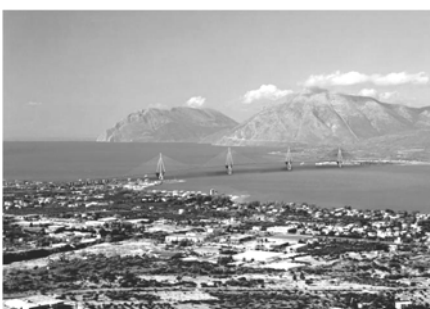
Figure 18 The 12 km long Rion-Antirion Bridge in Greece. The main bridge and its approaches were protected by SVPC devices manufactures in Italy (including 188 VDs).
