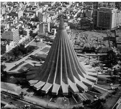
Figure 17 Madonna delle Lacrime Sanctuary at Syracuse (seismic zone 2), which may contain up to 11,000 persons, retrofitted by uplifting the dome (22,000 tons) and replacing the previously existing rubber supports by EPDs in 2006.
