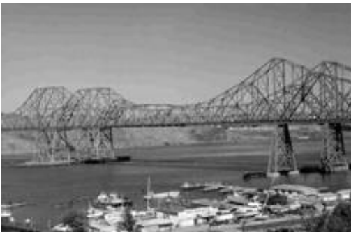
Figure 19 Carquinez Bridge , California (USA), retrofitted with STUs manufactured in Italy (centre, above).
