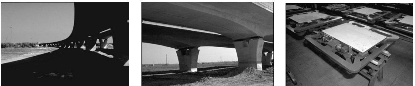
Figure 3 Coltano (former Mortaiolo) Viaduct of the Genoa-Rosignano freeway, protected by EPDs, rubber bearings (RBs) and STUs in 1990.
