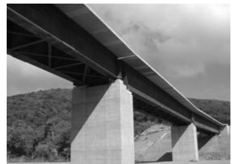
Figure 22 Caracas – Tuy Medio Railway in Venezuela (26 viaducts, overall length = 7,8 m, 217 isostatic spans), with over 1500 Italian SI/ED devices (centre, below) in 1999-2003.
