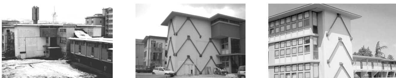
Figure 8 Gentile Fermi School at Fabriano (Ancona, seismic zone 2), an example of rationalist architecture, damaged after the 1997-98 Marche and Umbria earthquake and with some static problems even previously (left); its structural and seismic improvement with Visco-Elastic Dampers (VEDs) in 2000 (centre and right).
