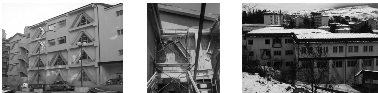
Figure 7 (a-b) Left and centre: Domiziano Viola School at Potenza (seismic zone 1), seismically improved in 2000 (similar to the La Vista School in 1999) and its dissipative braces with EPDs. (c) Right: Giacomo Leopardi School , again at Potenza, seismically improved with the same system in 2004.
