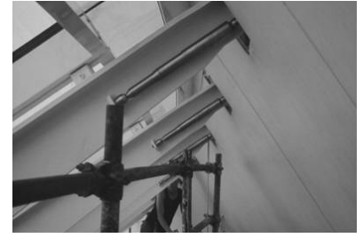
Figure 16 The new Dives in Misericordia Church , erected in Rome (seismic zone 3) in 2003, first application of the SVPC systems to new Italian churches, and some of the 32 VDs that were installed in the church to ensure the adequate seismic protection of this quite an irregular structure.
