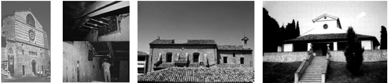
Figure 12 Further ancient churches retrofitted with SMADs. From left to right: (a-b) San Feliciano Cathedral at Foligno (Perugia, seismic zone 1), damaged by the 1997-98 earthquake (with view of its SMADs); (c) San Serafino Church at Montegranaro (Ascoli Piceno), damaged by the same earthquake; (d) San Pietro Church at Feletto (Treviso), also damaged by a significant earthquake in the past.
