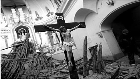
Figure 15 Church at Pisco (Peru) severely damaged by the earthquake of August 15, 2007. Most victims were due to the collapse of churches, similar to other events in other countries.
