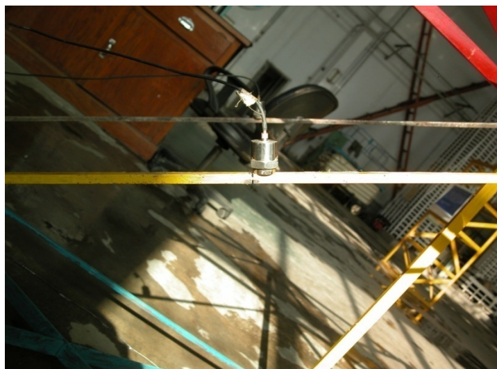
Photo 2 Accelerometer is attached perpendicularly to the middle of the member
