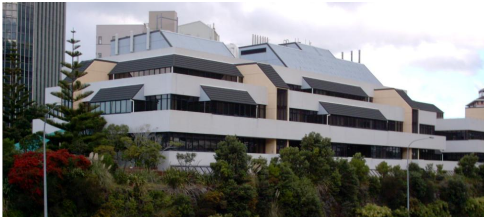
Figure 4 New Zealand's first base isolated building – the William Clayton building
