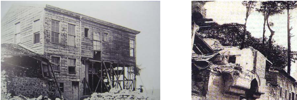
Figure 1. Damage in the 10 July 1894 Earthquake
