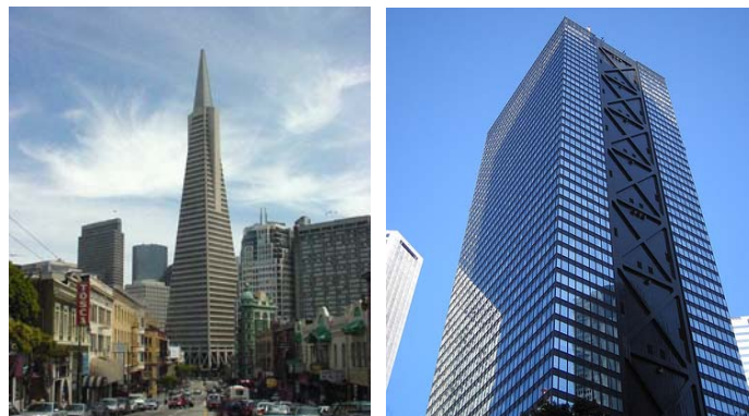
Figure 4 Morphology for earthquake resistance: Transamerica Building in San Francisco (William Pereira); Mitsui Building, Tokyo (Nihon Sekkei)
