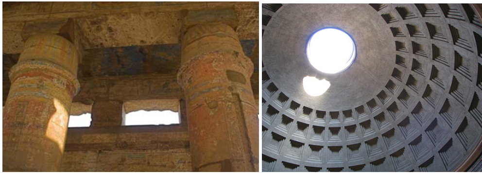
Figure 2 Vertical load carrying spanning structures. Architraves of the Temple of Karnak, Luxor, Egypt. Vault of the Pantheon dome, Rome.
