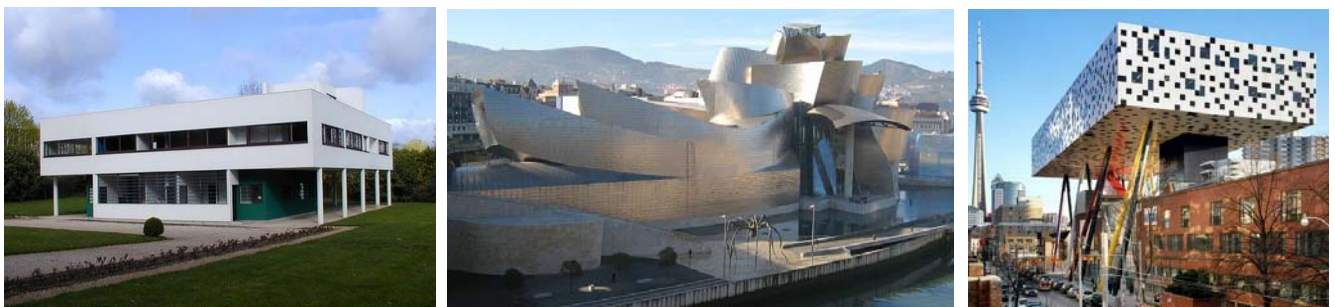
Figure 3 Vertical load carrying modern free-shaped buildings. Villa Savoye (Le Corbusier); Museo Guggenheim Bilbao (Frank Gehry); Toronto Sharp Centre for Design (Will Alsop)
