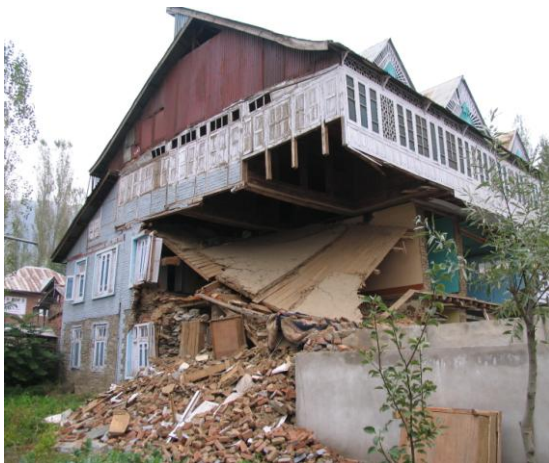
Figure 1 a) A building on slope failed due to excessive torsion during 2005 Kashmir earthquake (photo courtesy: Prof. C.V.R.Murty) . b) Failure of buildings due to settlement caused by seismic liquefaction during 1964 Niigata earthquake (NISEE).
