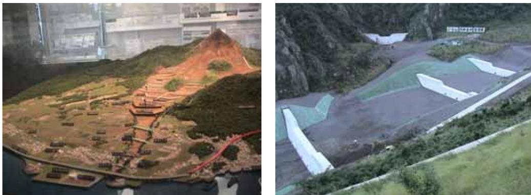
Photograph 3 Sand-trap dam constructed after the 1990s pyroclastic flow, Nagasaki
