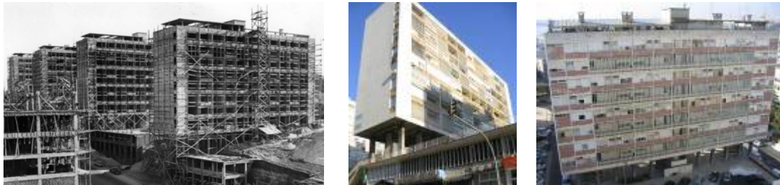
Figure 1. General views of the building block under analysis.
