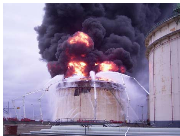
Figure 3 Tank fire occurred after two days of the event (photo by Fire and Disaster Management Agency)
