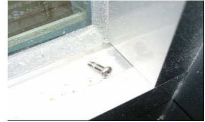
(b) Disengagement of height adjust bolt of transom
