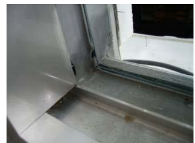
(c) Separation of a sealing member
